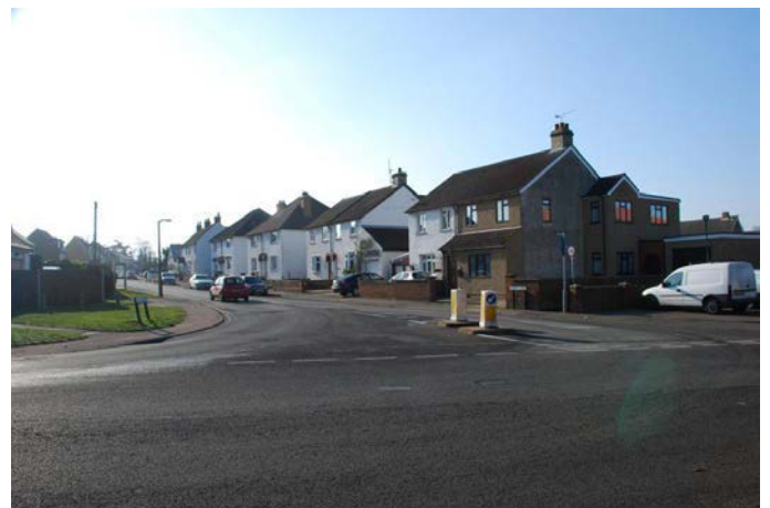
House Lane linear development
