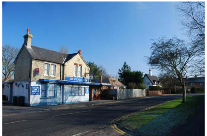
Cream brick Victorian pub (vacant)
